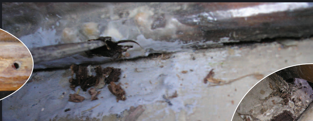
Below and left Parts of the wood were sodden and rotten through – see the black areas. Patches of good wood only spread the problem.
