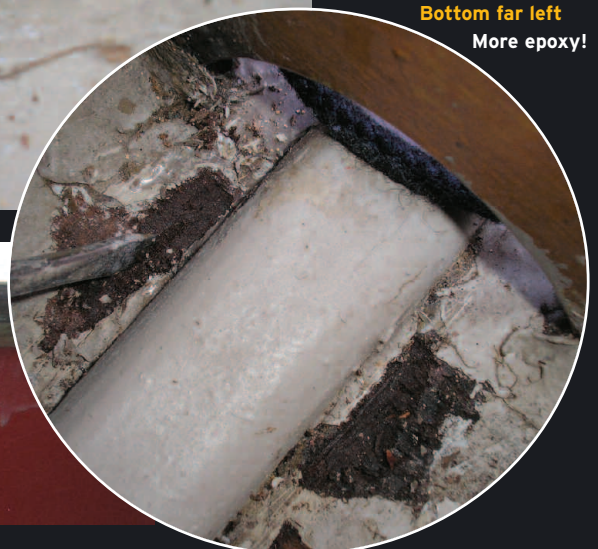
Below and left Parts of the wood were sodden and rotten through – see the black areas. Patches of good wood only spread the problem.
